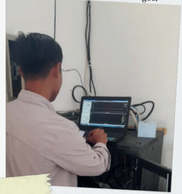
Inspeksi Site Transportable Boven Digoel
